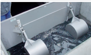
HydroStyx® discharge brake with controlled bottom outlet
